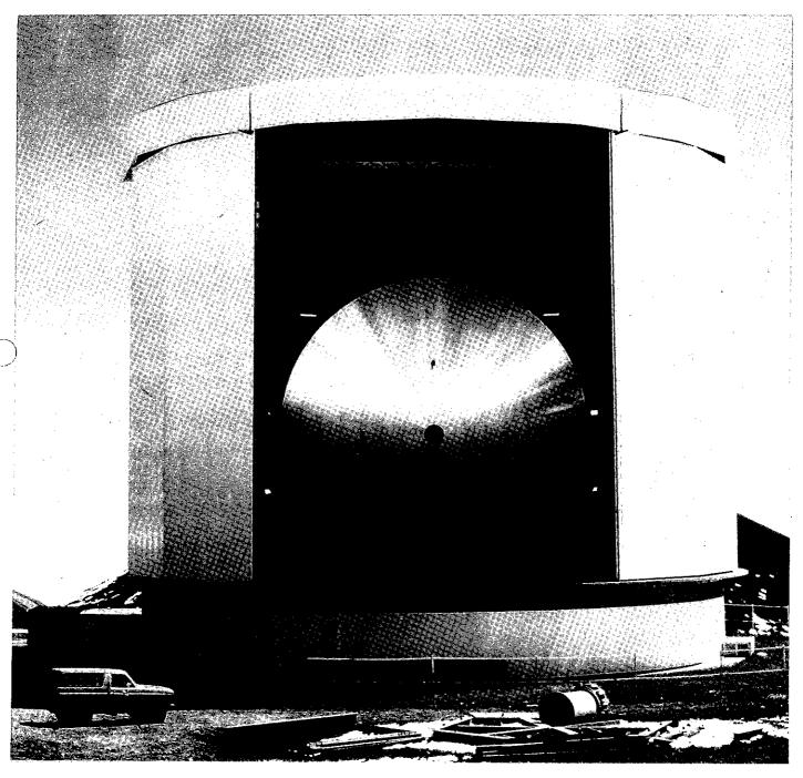
The front page of the previous issue of PROTOSTAR carried a photograph of the JCMT carousel with the membrane in position. The above photograph reveals the telescope that the membrane protects. At the time of the photograph the quadrapod that supports the secondary mirror was not in place.
