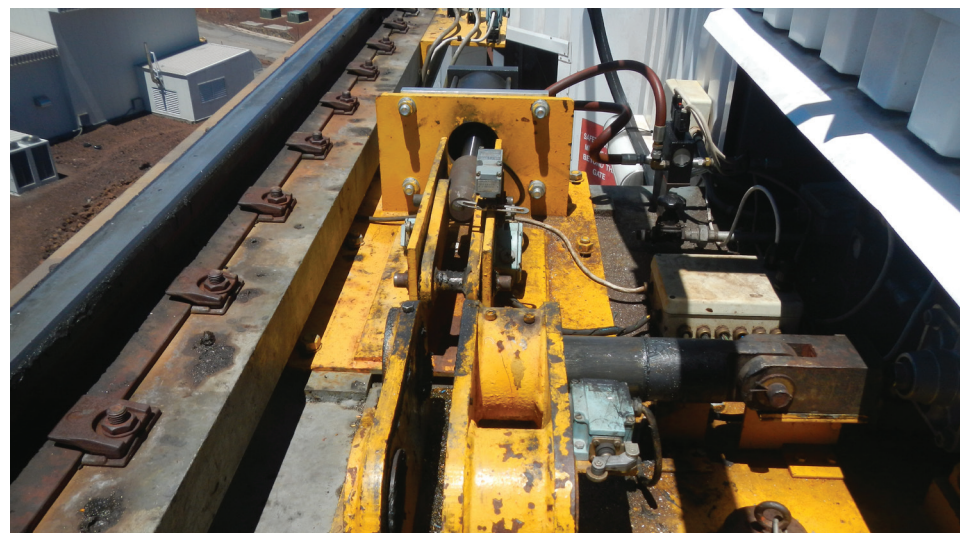
Figure 18: As the motors close the roof, this device slows the motors then grabs and pulls the roof fully closed. At the end of a cycle a locking pin is inserted with pneumatics.
