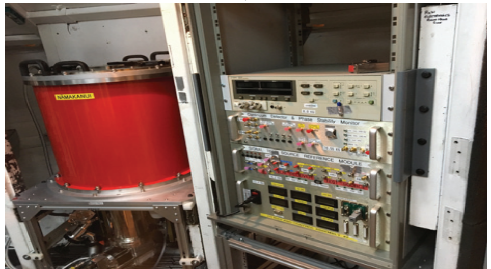
Figure 23: Nāmakanui is set up in the receiver cabin and ready for a performance test.
